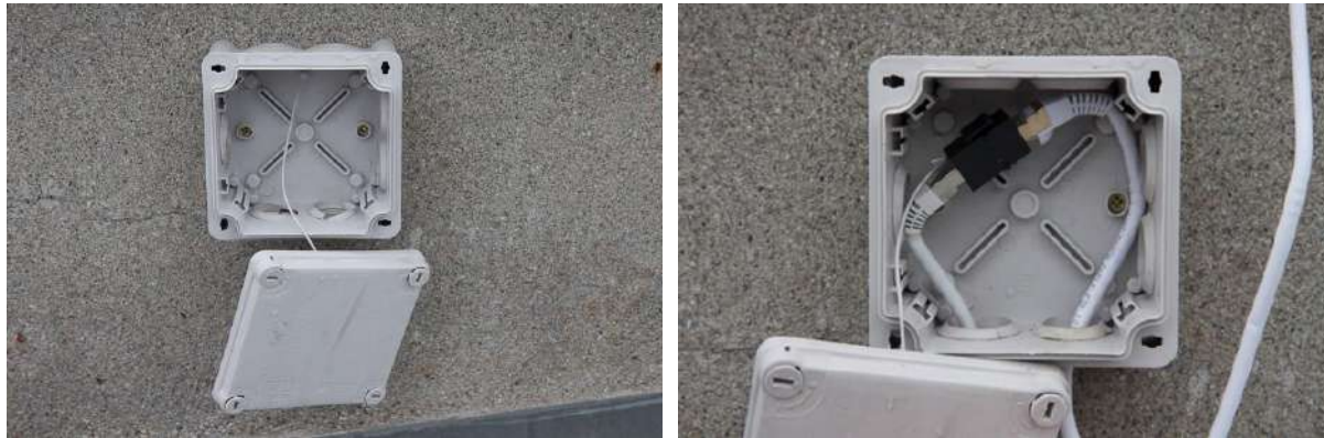
Figure 21 – Pictures of a correct installation of the junction box (B6) provided in the StAnD Meteor Camera Kit to extend the 5 m Ethernet cable with a second one. The junction box has to be installed vertically and the cables are to be inserted from the bottom holes, to avoid water infiltration. Credits: FRIPON - link
